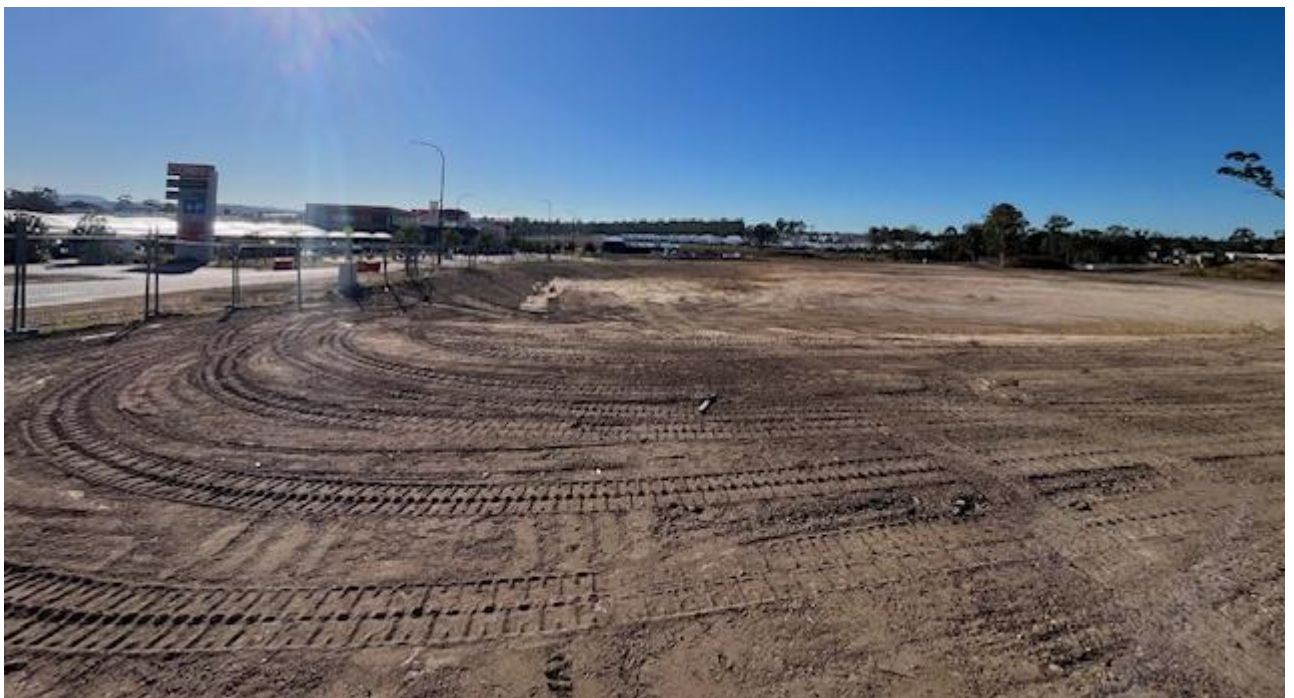
Figure 9: Looking East at the site from Bakehouse Road
