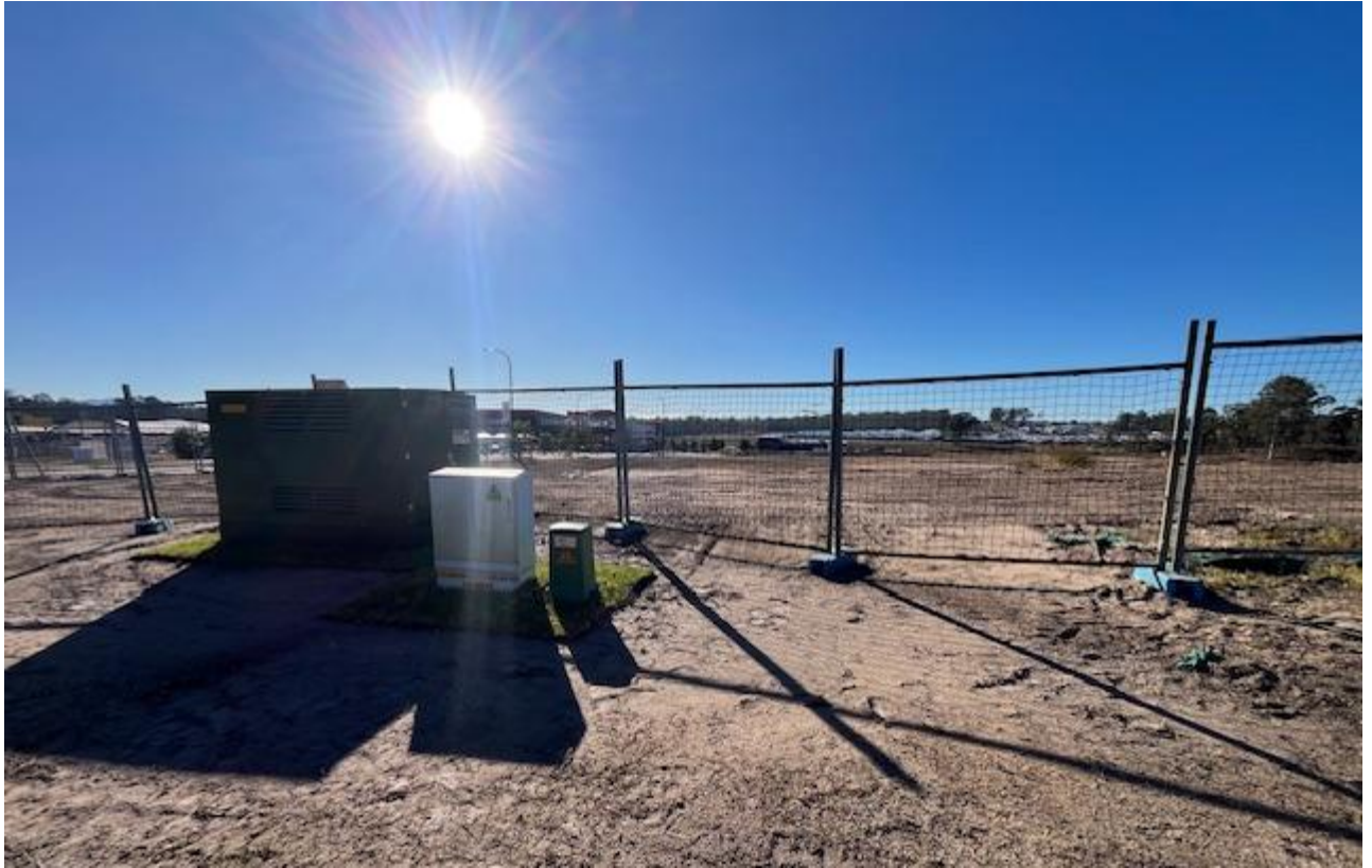
Figure 10: Existing substation on Bakehouse Road
