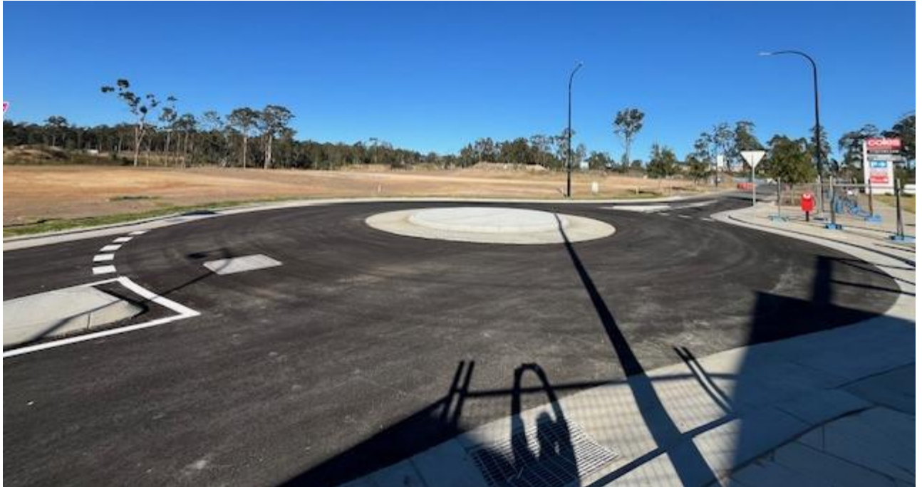
Figure 6: Looking South-west at the site from Empire Lane (new roundabout)
